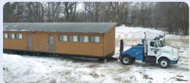
The first portable gets moved into place.
